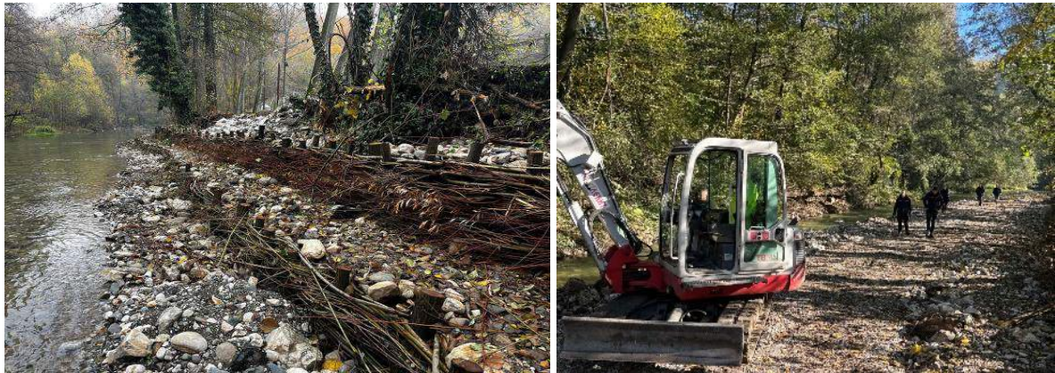
Willow wattle construction and sediment removal in Landscape of Exceptional Features Gradac River Gorge
