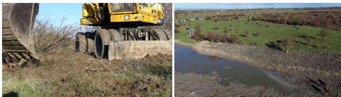
Removal of invasive plant species and construction of a shallow water-logged depression in Special Nature Reserve Zasavica
