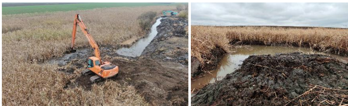
Dredging works in SNR Kraljevac revitalizing the critical wetland habitat for the European mudminnow and other endangered wildlienema
