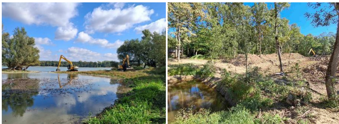
Dredging of canals for revitalizing wetland habitats in Special Nature Reserves Koviljsko-Petrovaradinski Rit and Obedska bara
